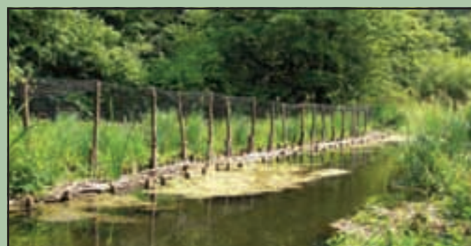
...and after work completed by EA, CMS and contractors
