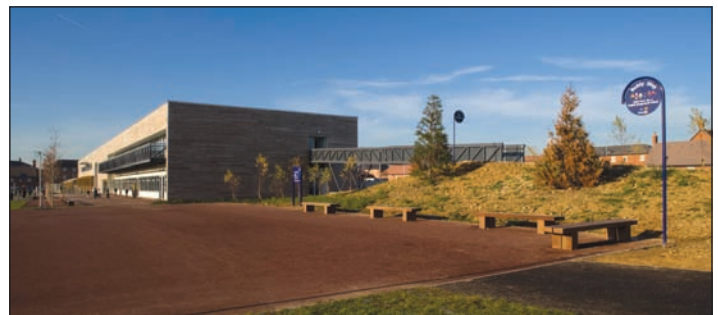
Hertfordshire's first eco-school, Howe Dell, was opened in 2007. A heatstore is located under its playground (above) whilst Photo Voltaic panels also provide electricity for the school (front cover).
